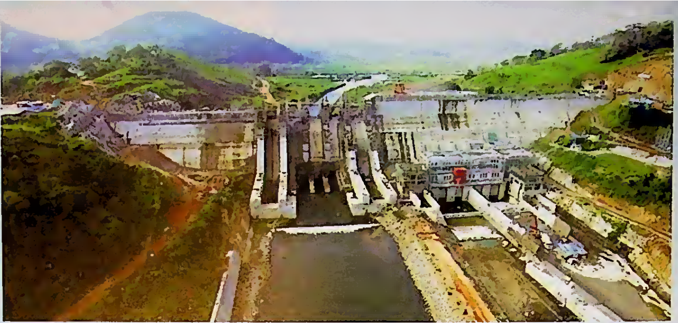
Moragahakanda - Kaluganga Dam
